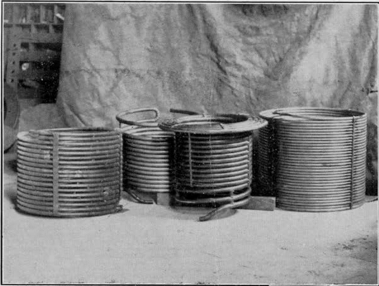
Fig. 4.—THE COILS OF THE LESLIE BOILER BEFORE ASSEMBLY. Although it does not show in the picture, the coil on the extreme left is made of finned tubing.
